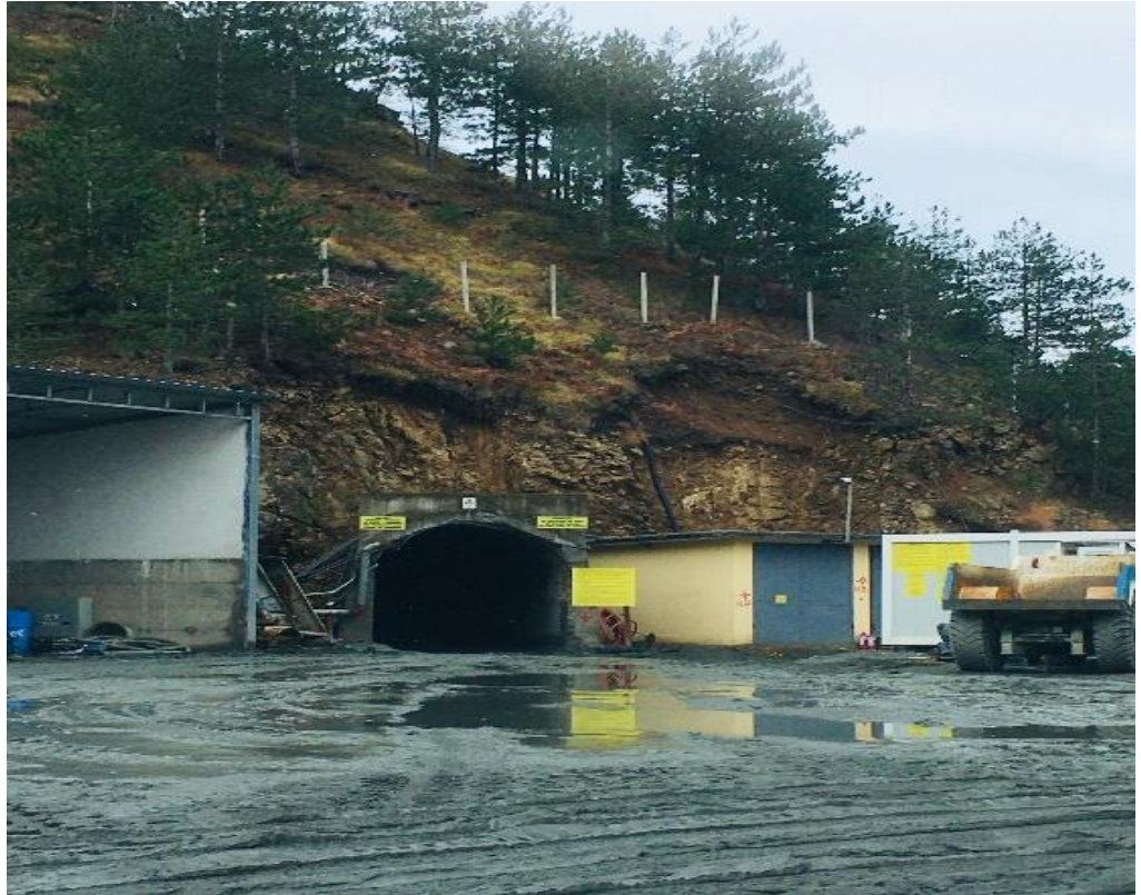
Fig No. 11 Main Ramp entrance Spaç Mine
