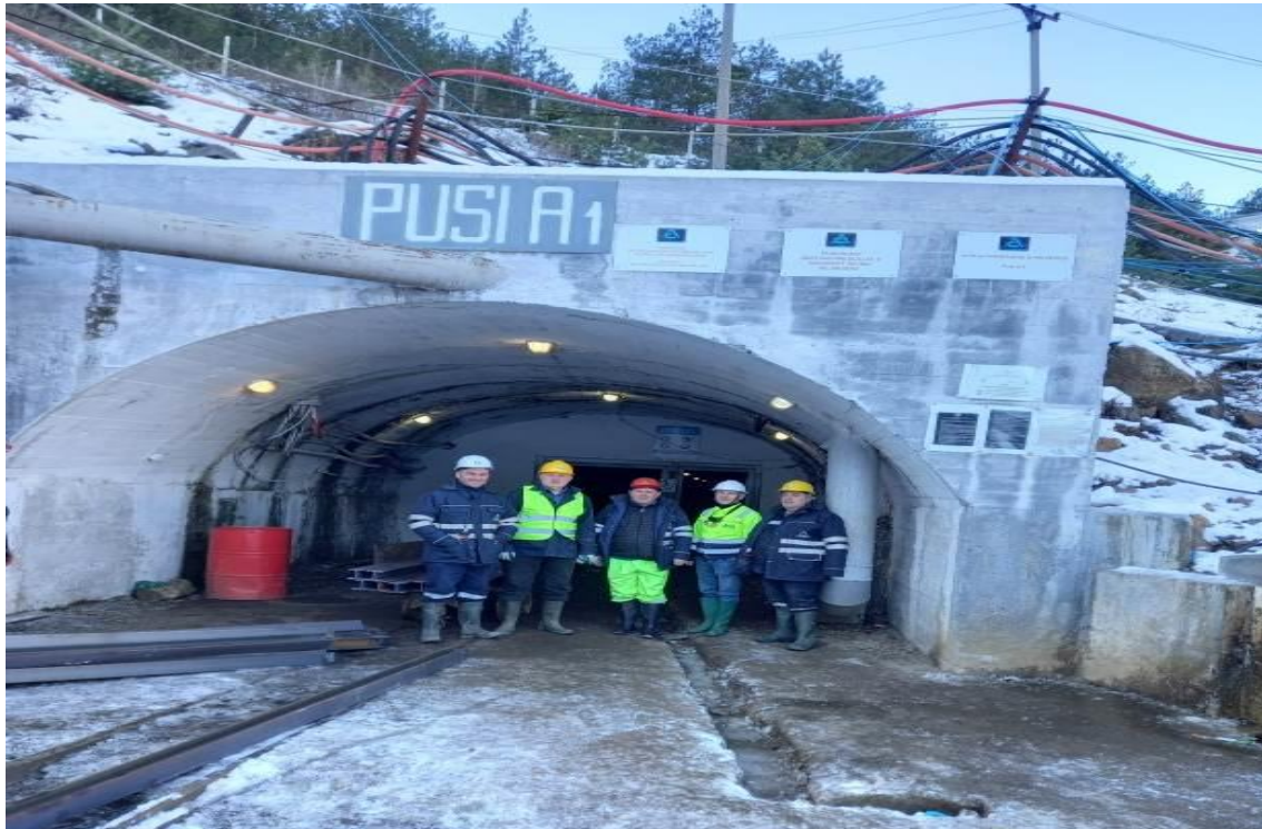
Fig No.6 Shaft A1 Entrance Bulqiza North
