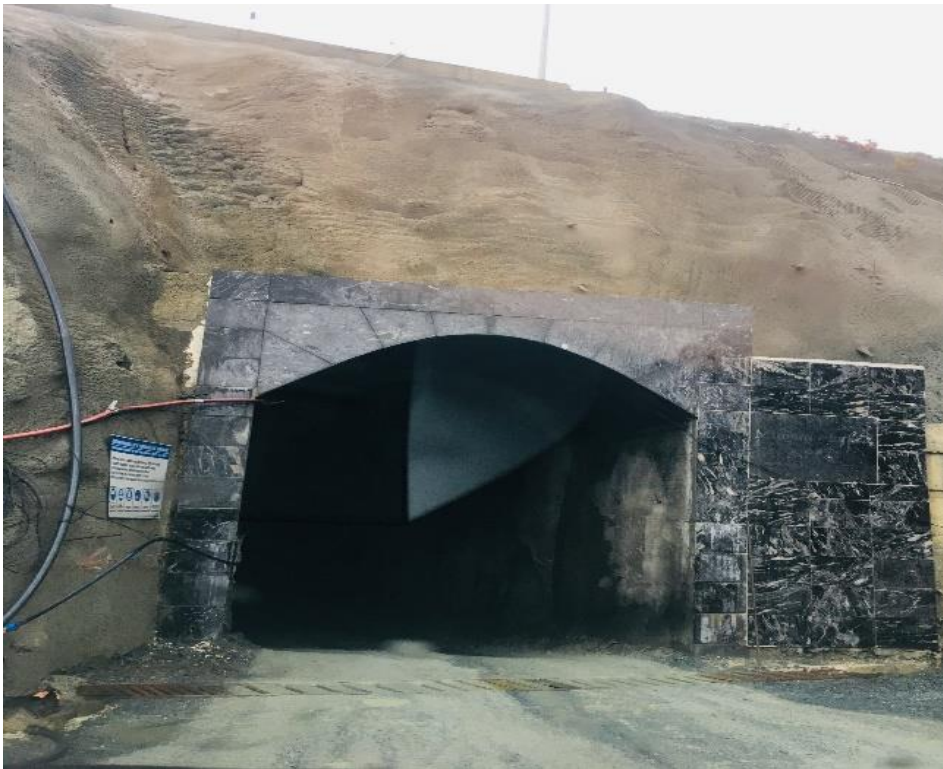
Fig No.12 Main Ramp entrance Munella Mine
